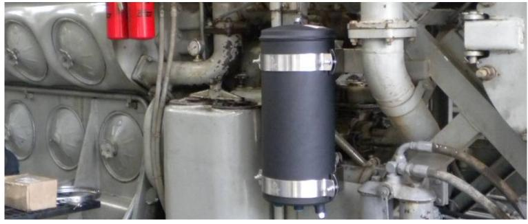
The WATER filter unit is installed on the external structure of the GENERAL MOTORS engine. Installation takes approximately 4 hours.
