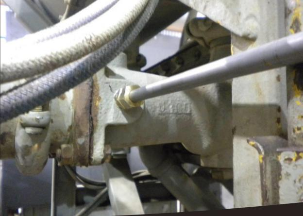
Return of the filtered water to the suction side of the pump
